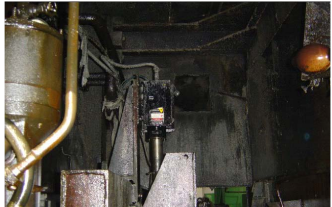
Exit of Cold Rolling Mill
