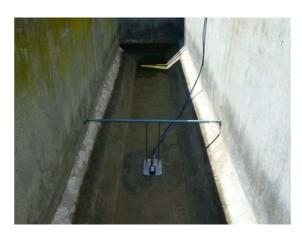
Anareobic stages of industrial WWTP have a very long retention time. Optimation of the process is performed by special analysers monitoring concentration of fetty acids and other compounds.
